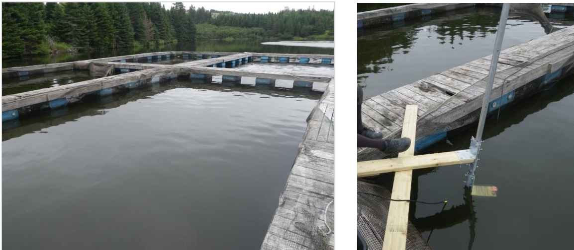
Figure 16. View of the netted pen and boardwalk structure on pond #2 at North River Fish Farms (Left). Preliminary positioning of the Gemini sonar on the pole mount (Right).
